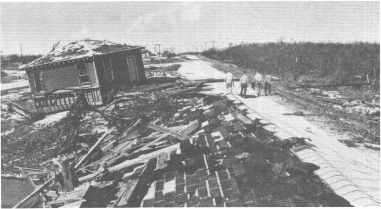
Though this house remained intact, the force of a coastal flood knocked it off its foundation, causing extensive damage.
