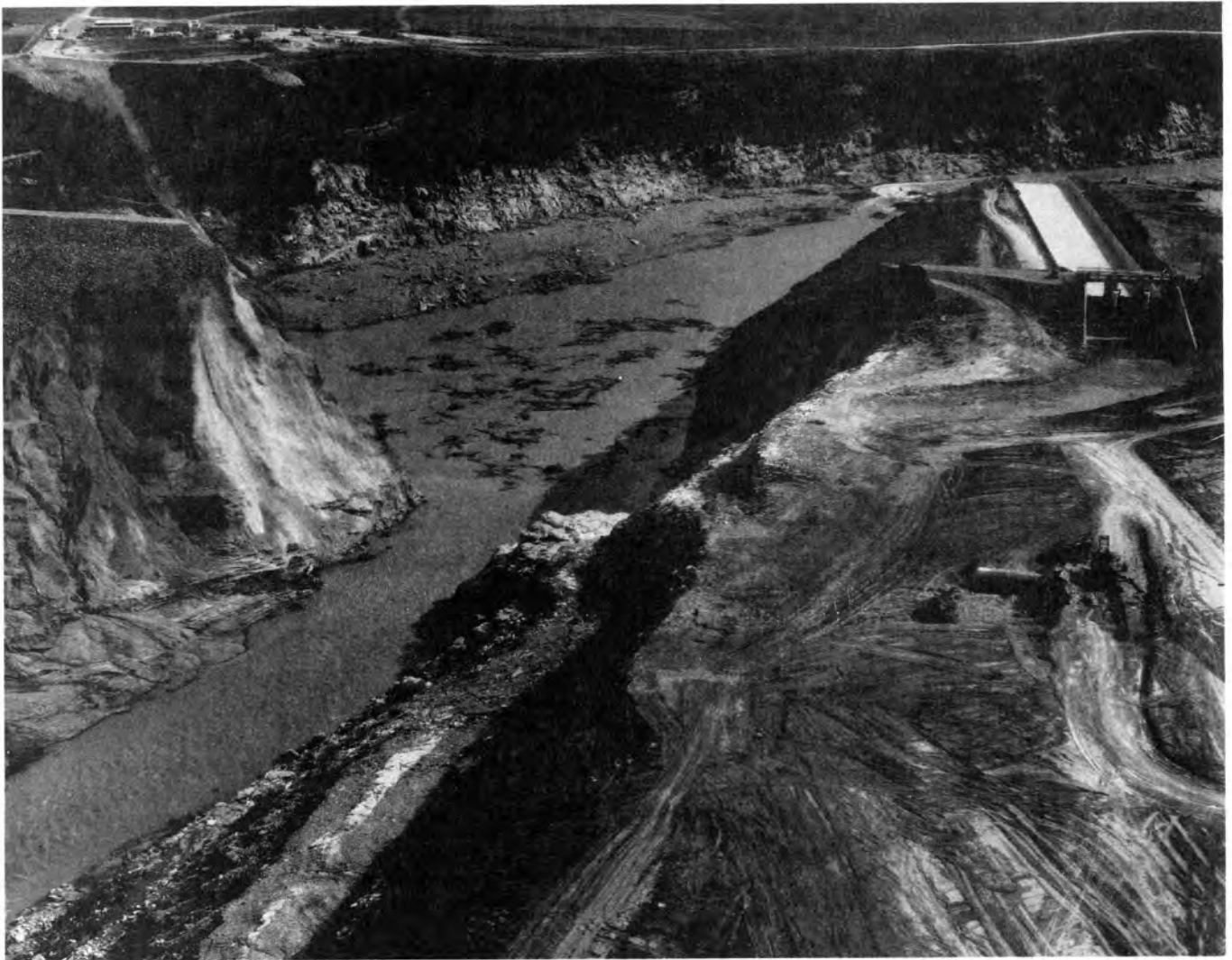
Figure 5-1. The Teton Dam, a Bureau of Reclamation project, collapsed in 1976 killing 11 people and causing millions of dollars in damages. The dam's collapse illustrated, once again, that structural solutions to flood problems are not without inherent risks.
