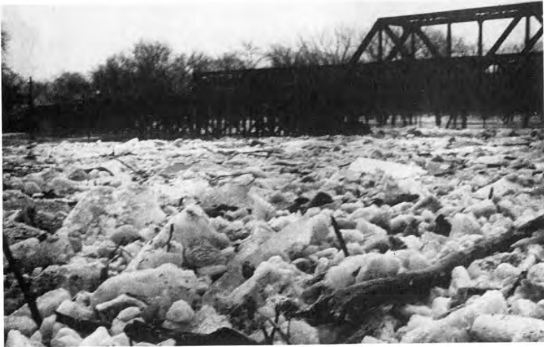
Figure 10-2. This railroad bridge is an example of a man-made structure that can restrict the flow of ice and debris and result in an ice jam. Source: St. Paul District, U.S. Army Corps of Engineers.
