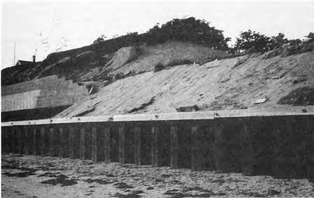
Figure 6-2. Shore erosion control structure in Massachusetts. Source: Jon Kusler.
