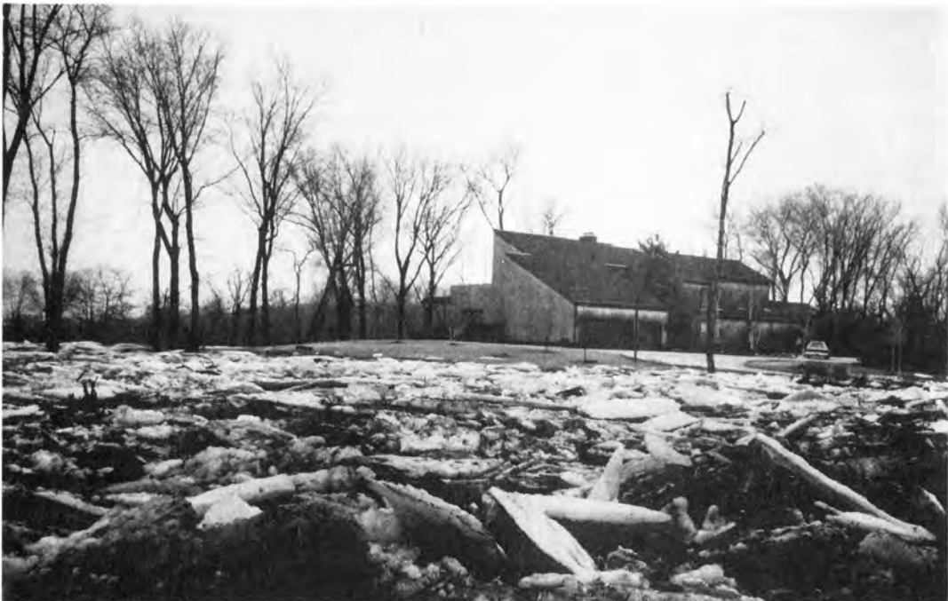
Figure 10-5. This house has been protected from flood and ice damage by being elevated on fill. Source: Mary Fran Myers.
