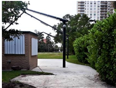
Approaching Utility Building
